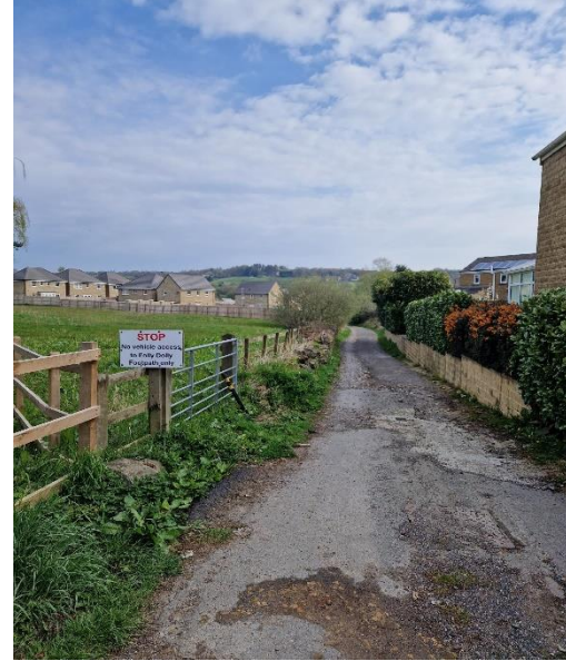
Photo 3: Application route leads north-north-easterly and narrows in width to approximately 3.5m. A sign adjacent the Application route states: 'STOP No vehicle access to Folly Dolly Footpath only'. The surface is poorly metalled and irregular.
